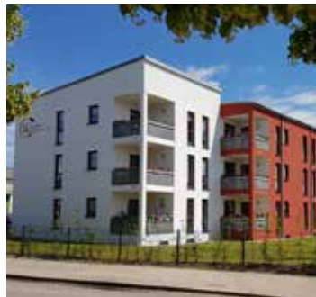
Neubau in Gägelow in 2016
